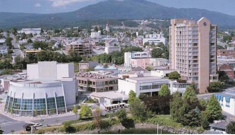
Vancouver Island Convention Centre, Nanaimo
